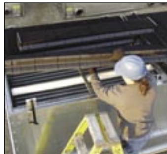
Inspecting drift eliminator.
